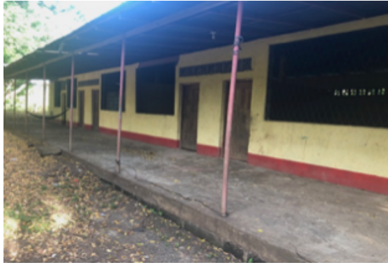
The separate premises to be upgraded
